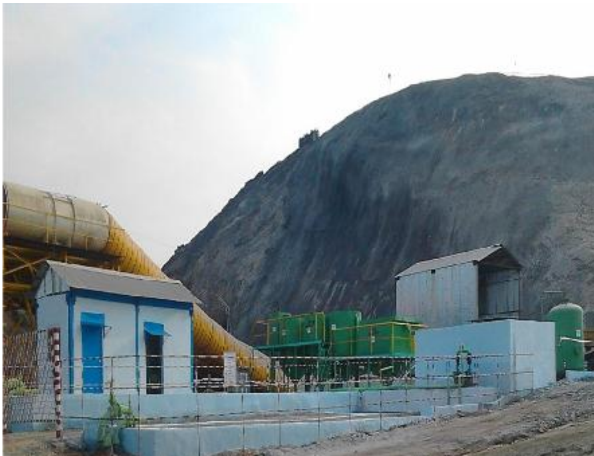
1 MLD WASTE WATER TREATMENT PLANT FOR ROCK CAVERN PROJECT. M/s. HINDUSTAN CONSTRUCTION COMPANY LTD, PADUR, KARNATAKA
