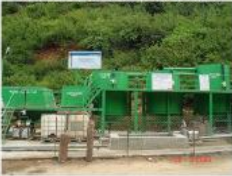
VIZAG CAVERN PROJECT (HCC) LOVA GARDENS VISAKHAPATNAM 1MLD WWTP
