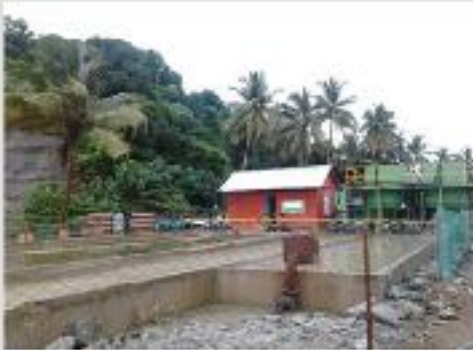
MANGALORE CAVERN PROJECT (HCC) KOT (IV) MANGALORE KARNATAKA 1MLD WWTP
